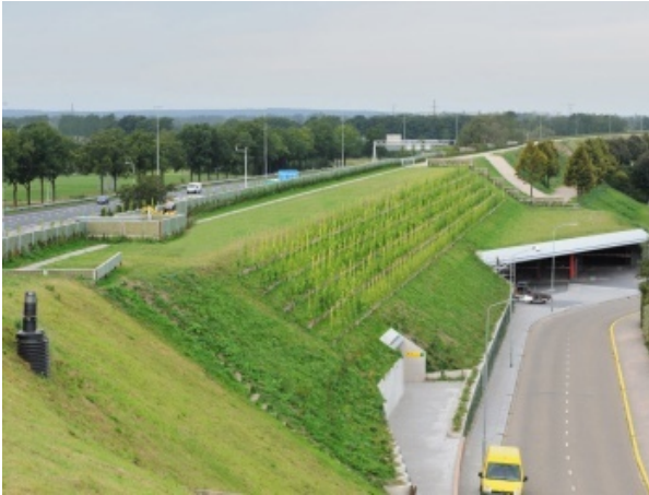
Figure 2.3: the parking garage of the CineMec in Ede is built into the noise barrier for the A12 motorway in the Netherlands
