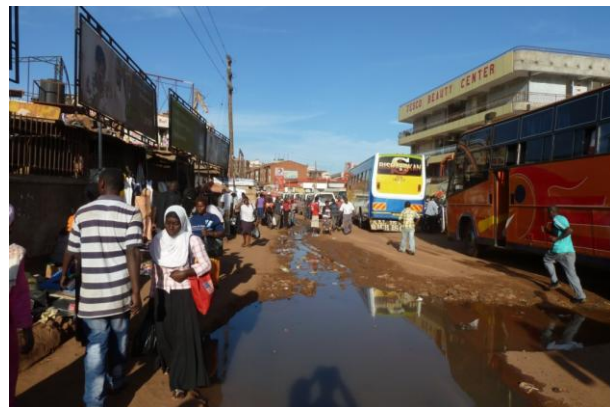
Figure 4-15: Poor drainage is a major issue
