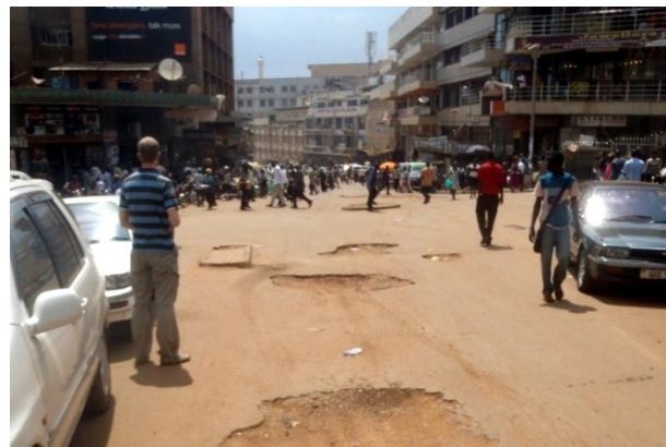
Figure 4-13: Potholes are common in the streets of Kampala
